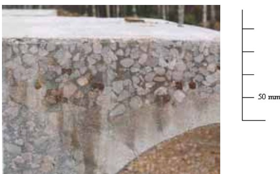
Fig. 4.6.5.19: The mock-up used for the repair trial has been cut in sections revealing the condition of the repair along the section tested. It can be seen that the first 150 mm is reasonably well formed with both aggregates and binder. There is however a layer of grout without aggregates, which corresponds with the “weak” layer suggested by SASW.
