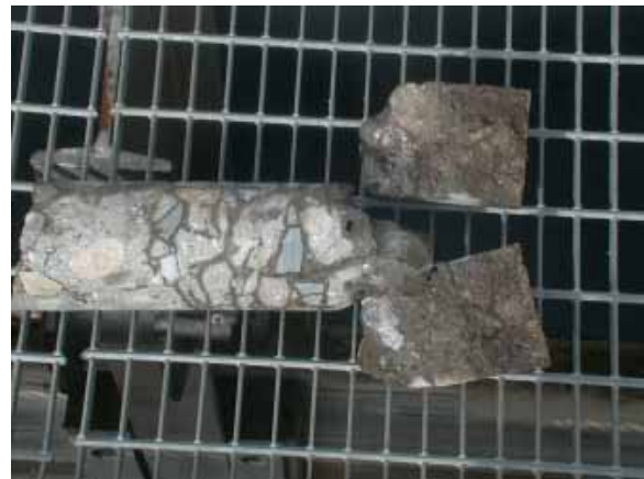
Fig. 4.6.5.1: Dam structure northern Sweden. Concrete cracking caused by ASR. The surface cracks are significant – running perpendicular to the concrete surface. The outer 100 mm has separated on drilling out. Internal cracks and porosity can be seen by the dark, moist pattern
