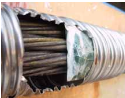
Fig. 4.3.7.9: Cable duct being prepared with air- and water-filled voids. The cable duct has a diameter of 70mm and contains 12 x 12.5 mm vsl cables, i.e. a heavily reinforced and congested cable duct. The “voids” are placed around and outside the cables. The duct was then cast in a 300 mm thick concrete beam
