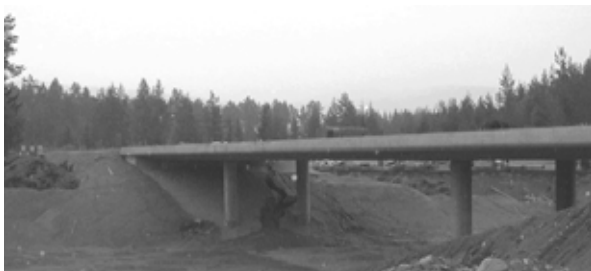
Fig. 4.2.10: Newly constructed bridge in Norway. The bridge slab is 850 mm thick and tapered at the edges. Some drying-shrinkage cracks appeared in the top surface. The w/c-ratio of the concrete is 0.4 and the maximum aggregates are 25 mm. The visibility of the back wall (underside of the bridge slab) tells us that the surface-opening cracks are probably shallow and that the concrete is otherwise free from internal damage. See Fig. 4.2.11.
