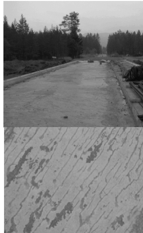
Fig. 2.5.2: A new bridge in Norway. Drying-shrinkage cracks appeared after casting the slab. The crack depths were found to be less than the cover thickness to reinforcing.
