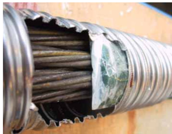
Fig. 3.5.7: Cable duct being prepared with air- and water-filled voids. The cable duct has a diameter of 70mm and contains 12 x 12.5 mm vsl cables. It is in other words a heavily reinforced and congested cable duct. The "voids" are placed on the outside of the cables. The duct was then cast in a 30 mm thick concrete beam.
