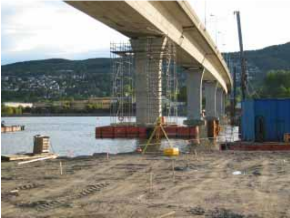
Fig. 2.4.1: A box-girder bridge in Norway. The pre-stressed cables in the beams are being examined using a Cobalt isotope and Betatron.
