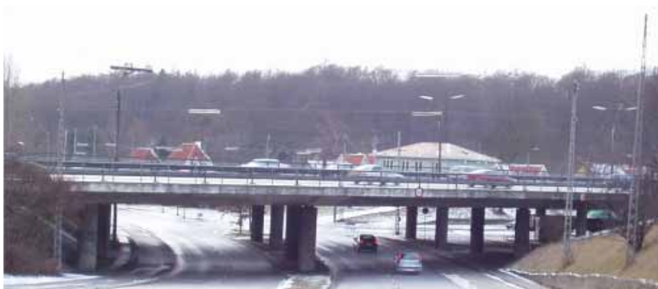
Fig. 3.5.10: Skovdiget bridge in Copenhagen. This 30, year old bridge has been suffering from frost damage, asr and reinforcement corrosion. Some of the post-tensioned beams were badly cracked.
